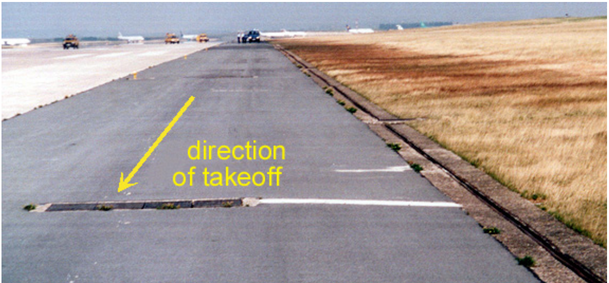
Figure 28: Burnt grass on the edge on the runway
